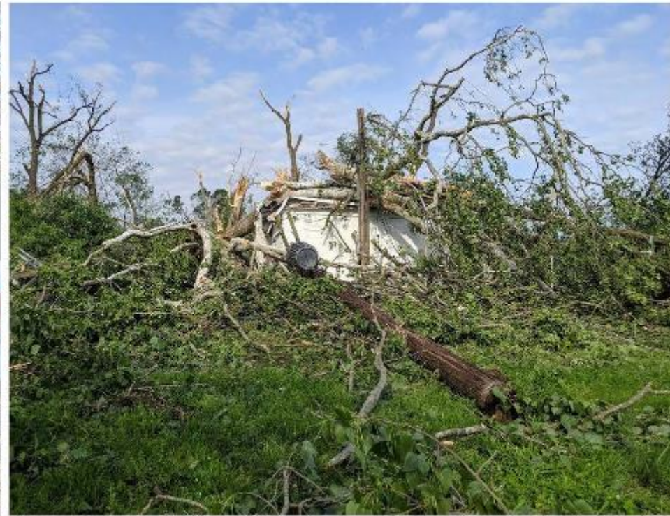
N-7 Stillwater Lift Station AFTER
