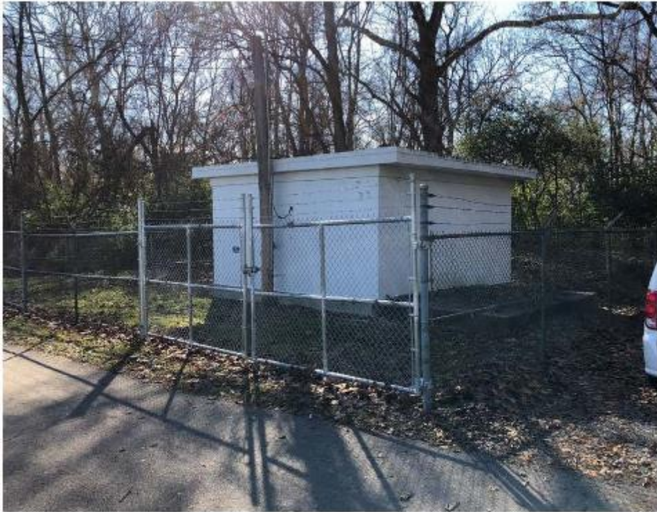
N-7 Stillwater Lift Station BEFORE
