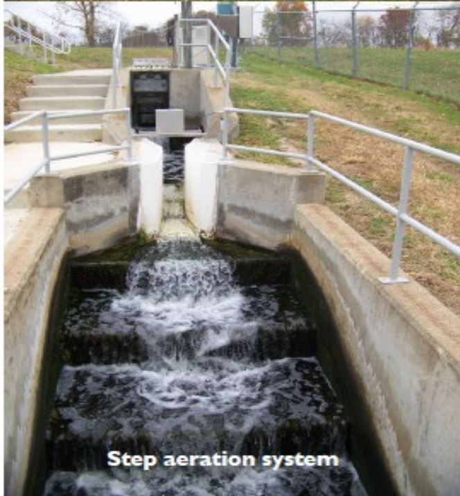
Effluent treatment structure
