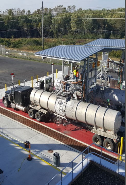
Biosolids land application facility (BLAF) in Columbus, OH
