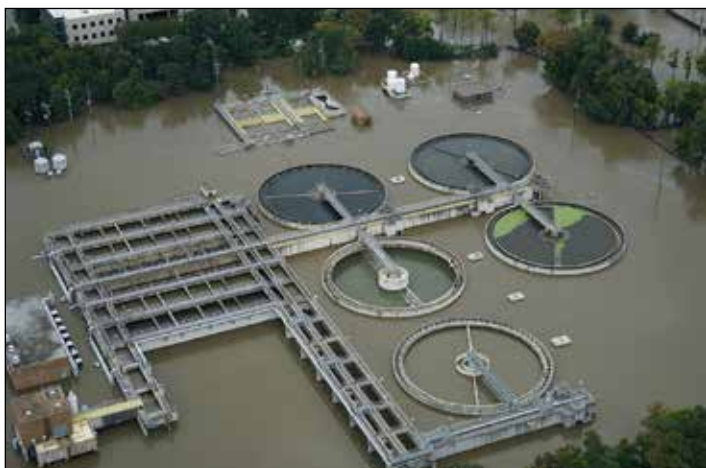
Flooded WWTP In Houston Texas Due to Hurricane Harvey Source: Texas A&M Transportation Authority
