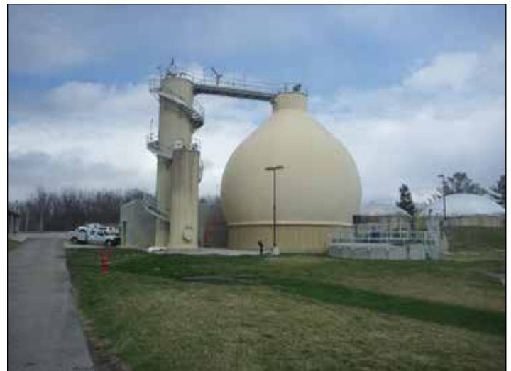
Egg Shaped Anaerobic Digester
