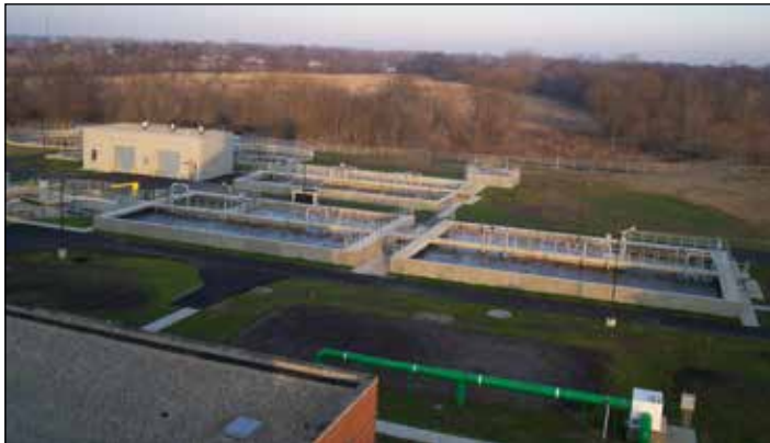
City of London Wastewater Treatment Plant.
