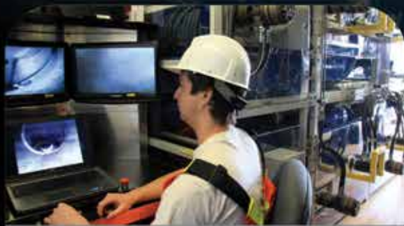
Totally Trenchless Lateral & Mainline Lining
