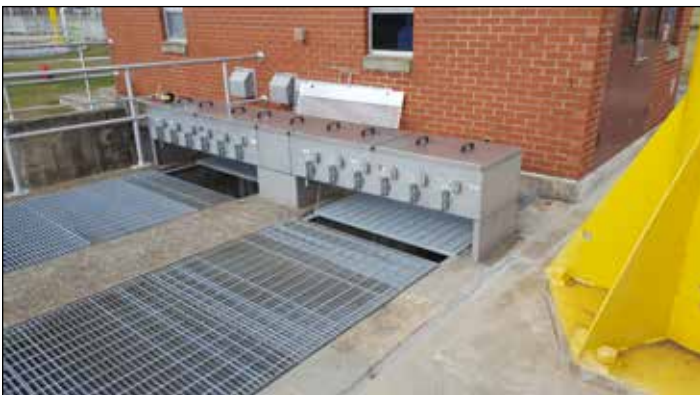
Ultraviolet Light Disinfection
