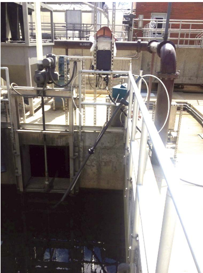
Figure 1: These pictures show the PVC pipe used as a pre-filter (Left) and the end of the pipe with the 1/8 inch holes and rag shield. (Right)
