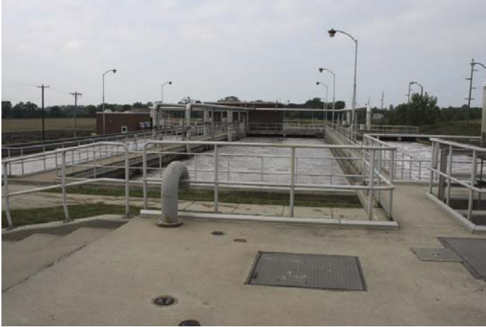
Extended aeration tanks
