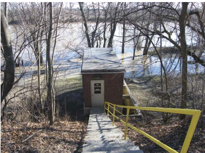
Lift Station Affected by RWI
