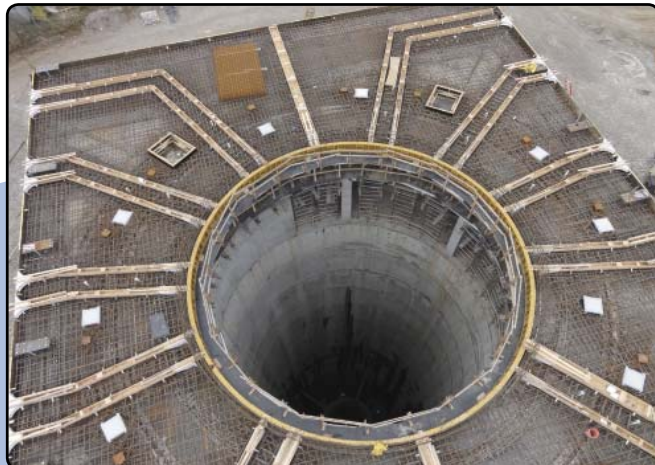
CITY OF COLUMBUS OARS TUNNEL ACCESS SHAFT
