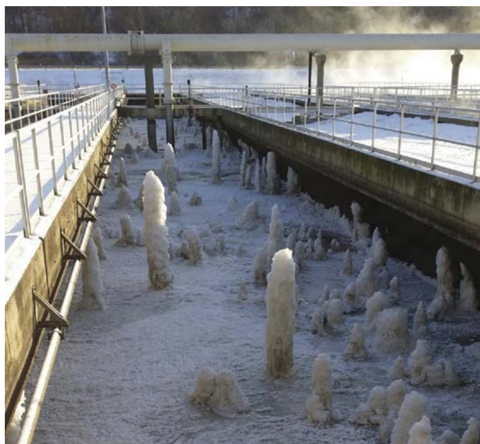
Photo by Southerly Wastewater Plant Operator Nick Fillipelli, NEORS These open-air aeration tanks inject air bubbles into the wastewater during the treatment process at the Southerly plant. As temperatures fell, nearing almost 40 degrees below zero with the wind chill, the surfaces froze, but water continued to bubble through holes in the ice.
