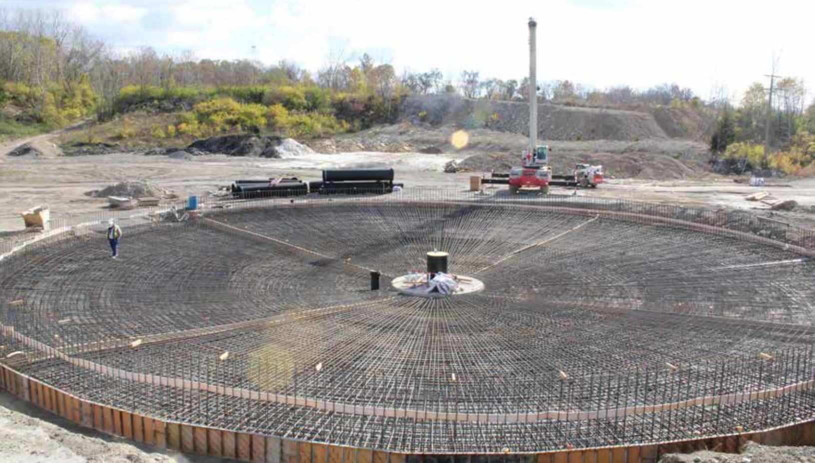
Final clarifier floor with 2 heavy rebar mats and 2 feet thick of concrete to be poured
