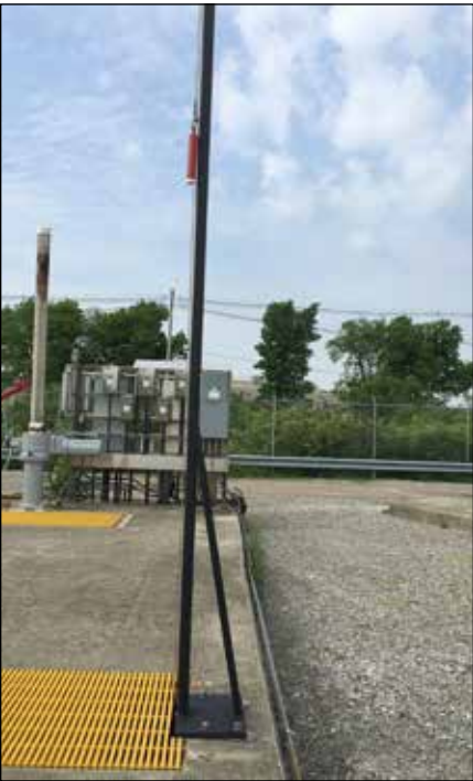
FDS Raw Sewage Level Indicator side view
