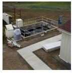
The Village of Creston's WWTP was upgraded in 2014 with improvements that included a new mechanical screen, raw pump and building improvements, an oxidation ditch, final settling tanks, blower improvements, auxiliary power, phosphorous removal and a new laboratory and administration building. This project also eliminated a tertiary filtration system. The design capacity of the treatment plant remained at 0.230 MGD on an average daily basis, with a peak design capacity of 0.800 MGD.
